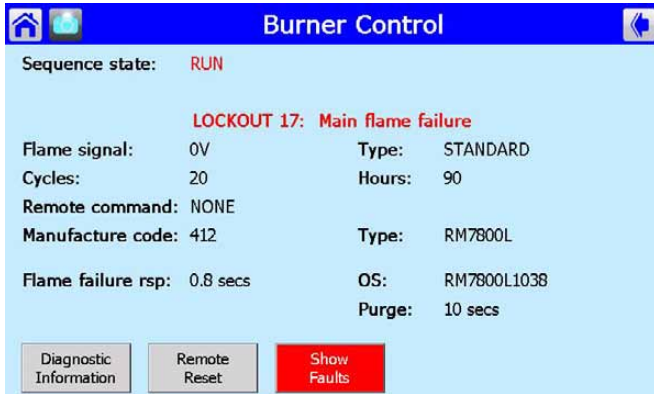
Fig. 77. Burner Control Status—Lockout.
