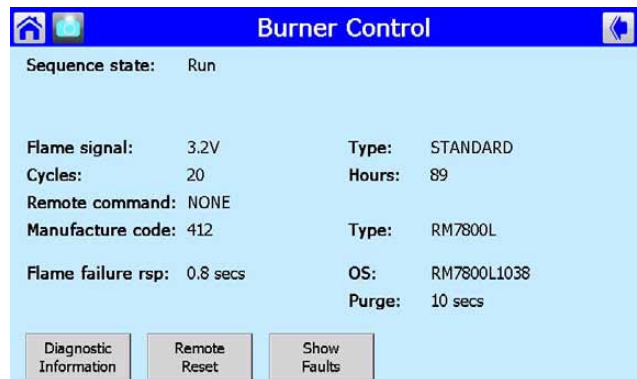
Fig. 76. Burner Control Status.
